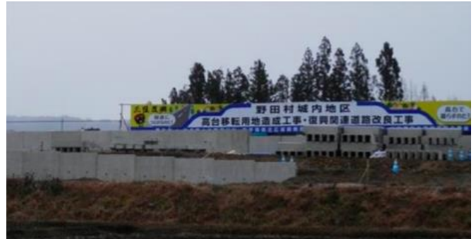
Nodamura new high group construction Reconstruction road construction
