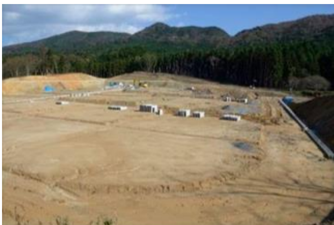
Current situation of Oshika Peninsula Kyubun Hama Residential development
