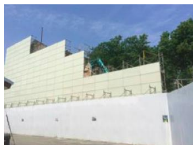
2014 - Ando Primary School demolition
