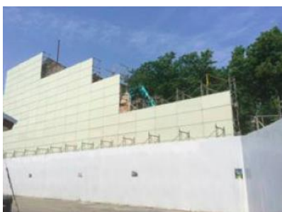
2014 - Ando Primary School demolition
