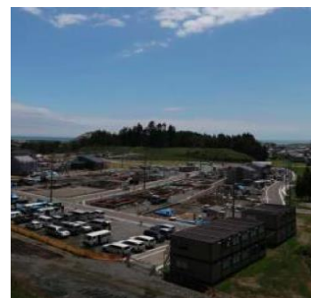
Jonai district high land Construction
