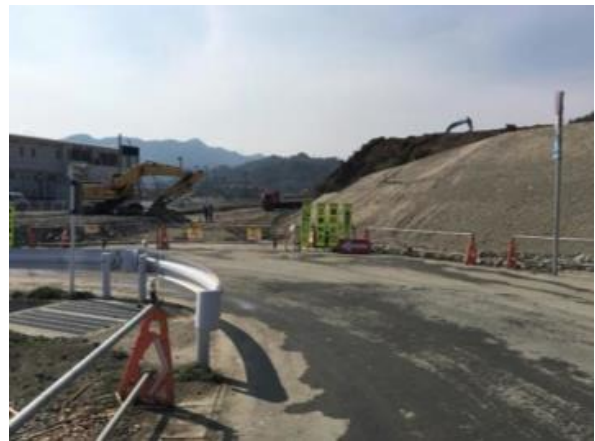
Levee Raising Construction still has a long way to completion
